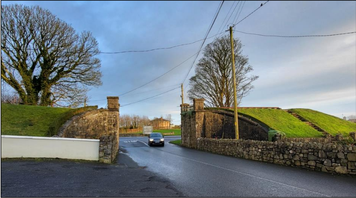
Figure 5.1.4.19d Former bridge along the previous L&NWR rail line
