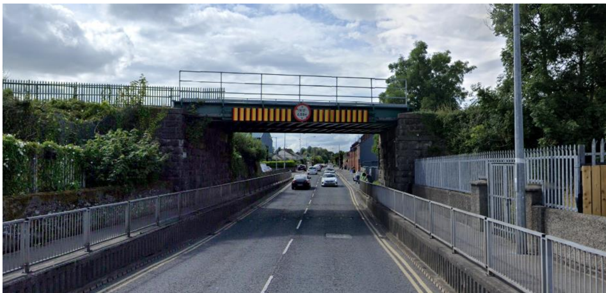
Figure 4.3.1 R934 in Dundalk looking west at Rail Bridge (Source: Google Maps)
