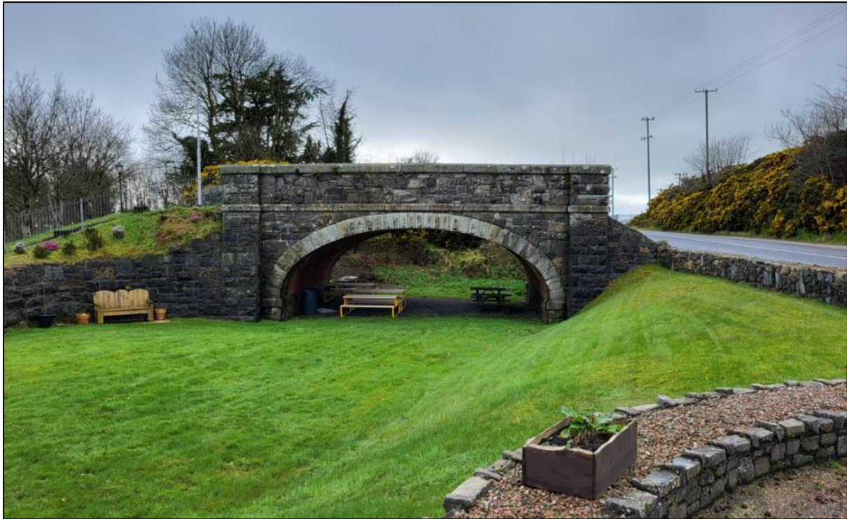
Figure 5.1.4.23b Decommissioned stone bridge crossing over the former L&NWR rail line, located in the direct vicinity of the quarry entrance
