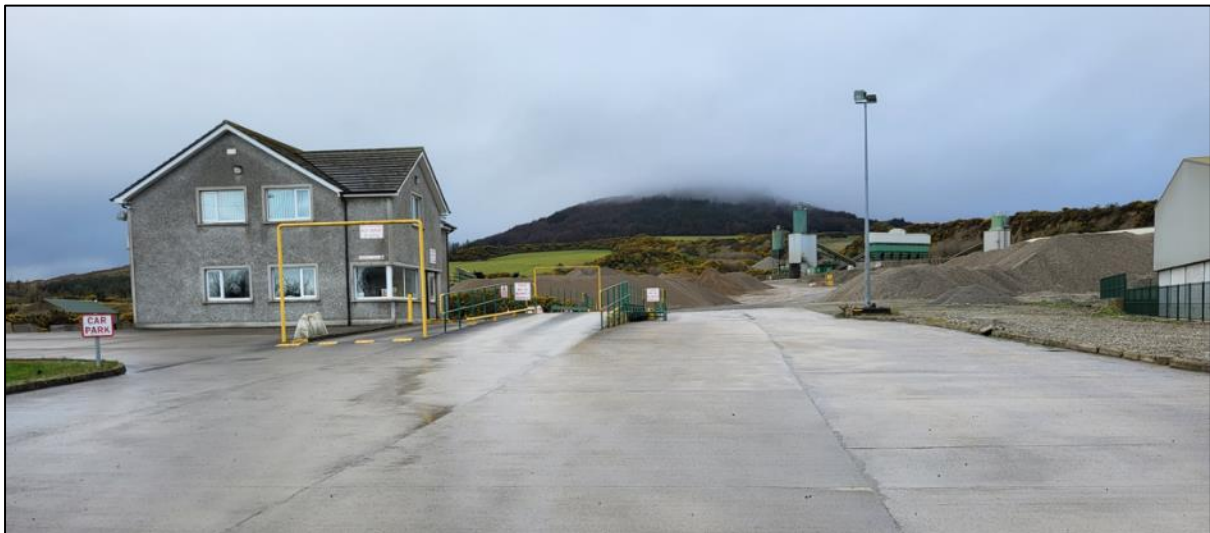
Figure 5.1.4.23a As with most quarries, the Ready Mixed Concrete Landscape Sub-Unit is an area of notably low landscape and visual value.
